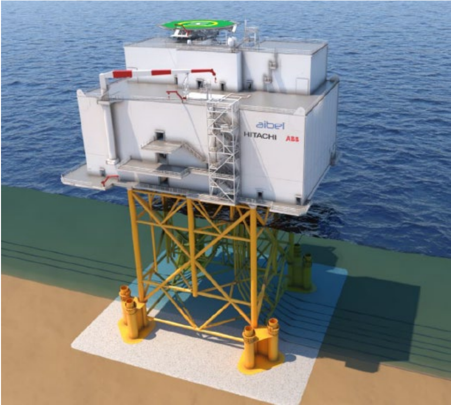
Figure II – 5. ILLUSTRATION OF A TYPICAL ESP, SHOWING THE OFFSHORE TRANSMISSION EQUIPMENT BEING SUPPORTED BY THE JACKET.
