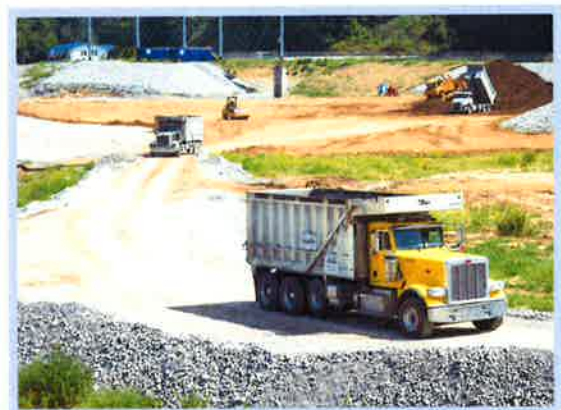
Workers finish a major project to relocate coal ash from close proximity to the Kentucky River to Smith Station.
