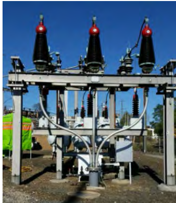
Figure 4– HPFF Termination (provided by PECO)
