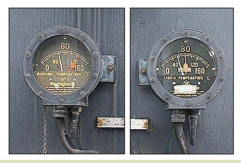
Illustrations of Analog Gauge Style Winding Temperature and Liquid Temperature Thermal Devices
